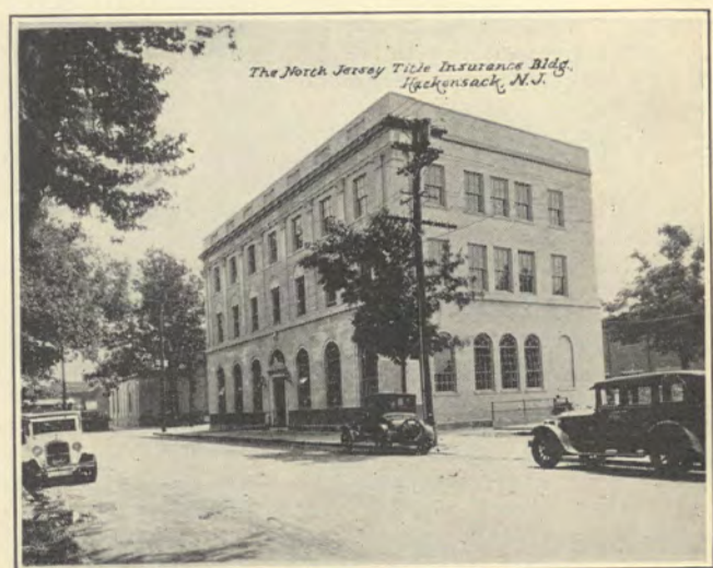
New home of North Jersey Title Insurance Co., Hackensack, N. J. The entire building is occupied by the company. It was especially designed to give every convenience and facility for the conduct of a title business and in addition a beautiful structure. The executive offices are on the first floor, closing rooms on second, and title plant on third.
