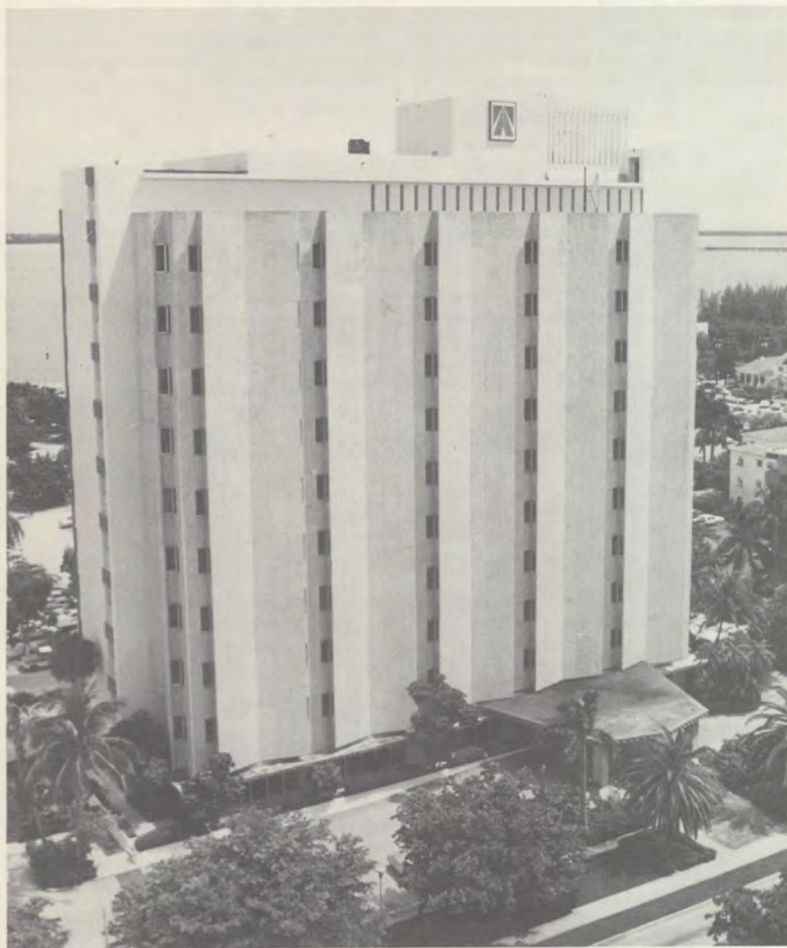
The former Aristar Building in Miami, Fla., now houses the American Title Insurance Co. home office staff and its Greater Miami Division—and has been renamed the American Title Building. The move represents the first of two for the company in Miami. The 150 Southeast Third Avenue office—formerly headquarters—will be remodeled and occupied by American's Miami Title and Abstract Division.
