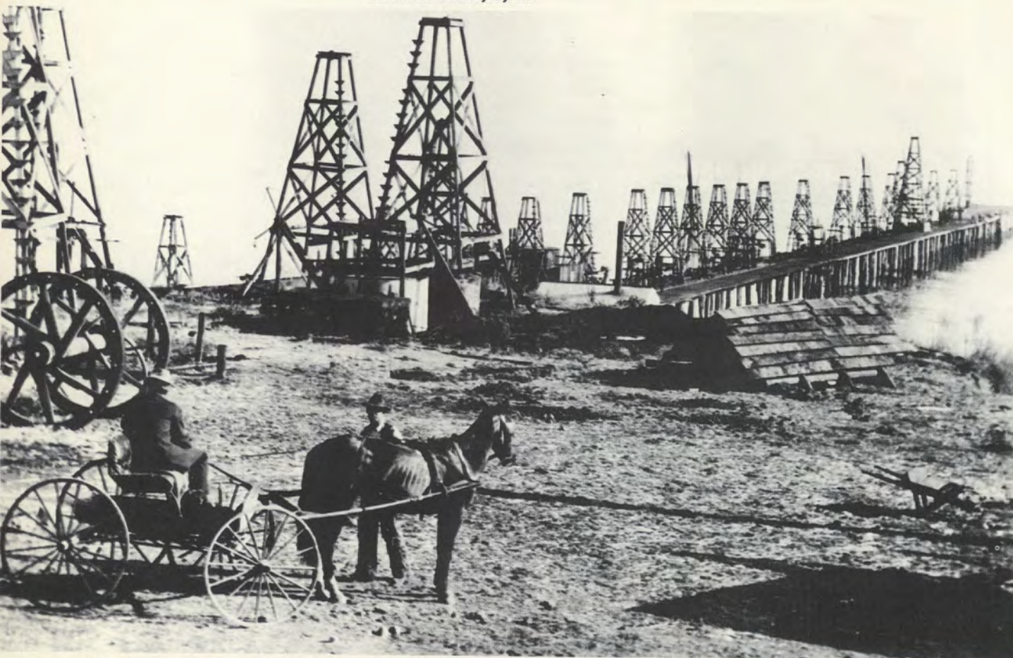
C.C. Pierce took this photograph of the Summerland oil field near Santa Barbara in 1902. They were the first oil wells drilled in the ocean. The Pierce Collection is the heart of the TI photo collection recently turned over to the California Historical Society.
