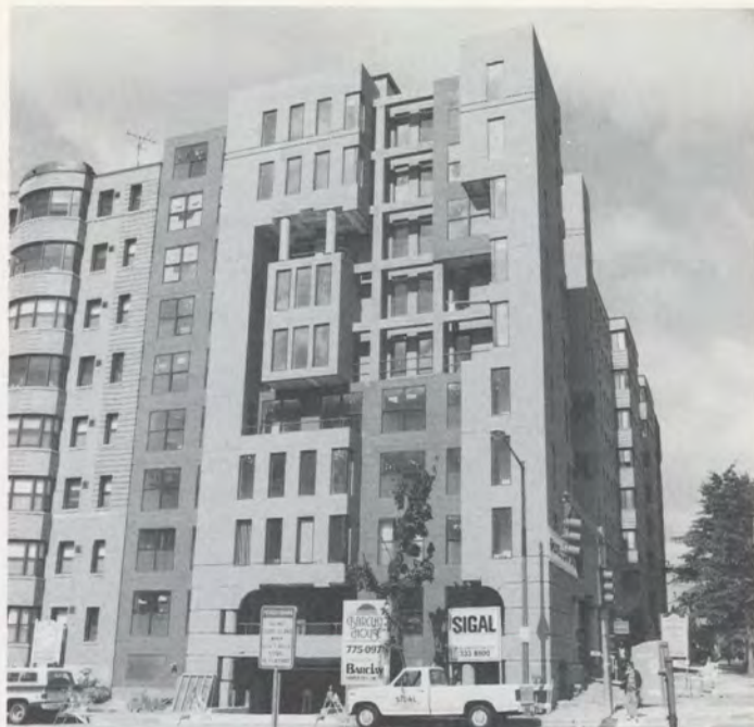
The Barclay House, the first urban timeshare project built in Washington, D.C., has 27 units owned primarily by businesses.
