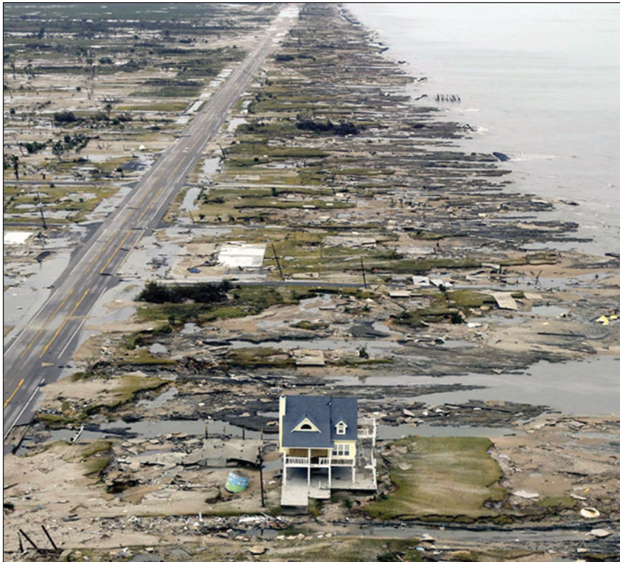
▲ Aftermath of Hurricane Ike in Galveston, TX
