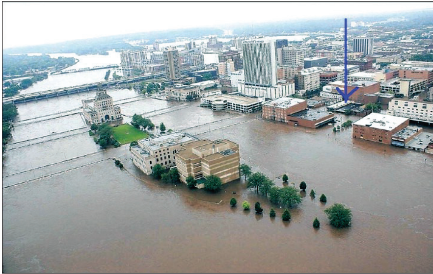
A Iowa Title Company, submerged to the roofline, in downtown Cedar Rapids.
